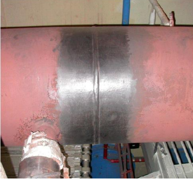
Fig. 3. Photo-documentation of circumferential weld on a pipe with limited accessibility.
