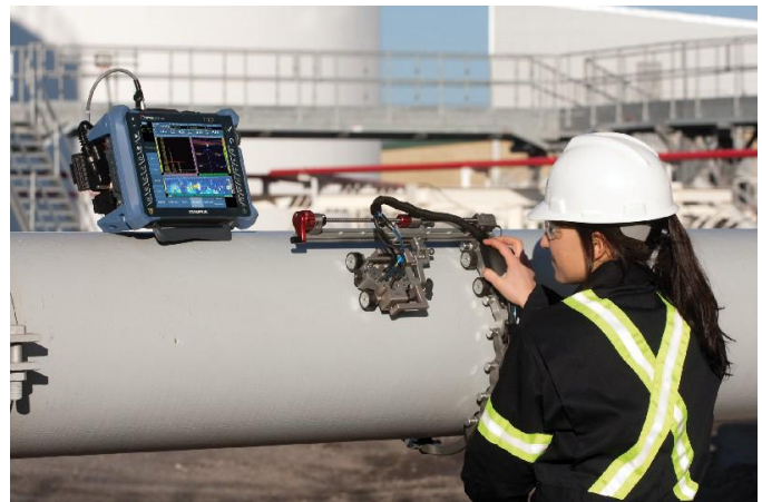
Fig. 1. Typical NDT setting for manual weld inspection.
