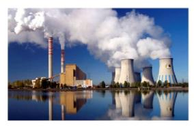
The **Belchatów Power Station** is a large 5298 MW lignite-fired power station situated near Belchatów in Łódź Voivodeship. It is the largest thermal power station in Europe, and fourth largest fossil fuel power stations in the world. Units: 12 x 370 MW 1 x 858 MW (supercritical)
