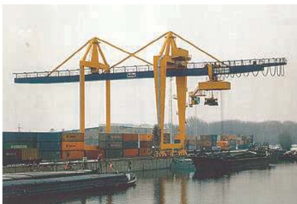
Figure 17.3.1: View of a portal-type loading crane
